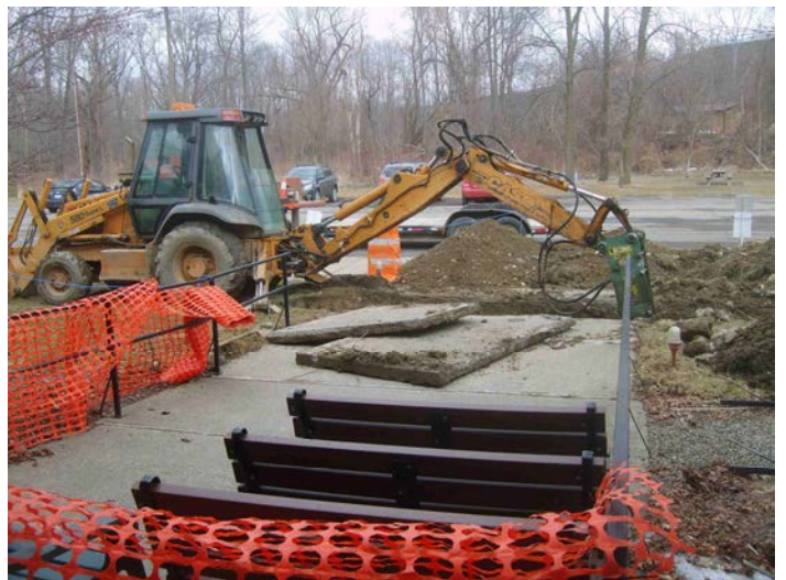
Kolo Excavating, hard at work on the waterline project
